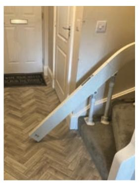
Where space is limited, or the stairlift rail would present an obstruction, our hinged rail is the ideal solution.
